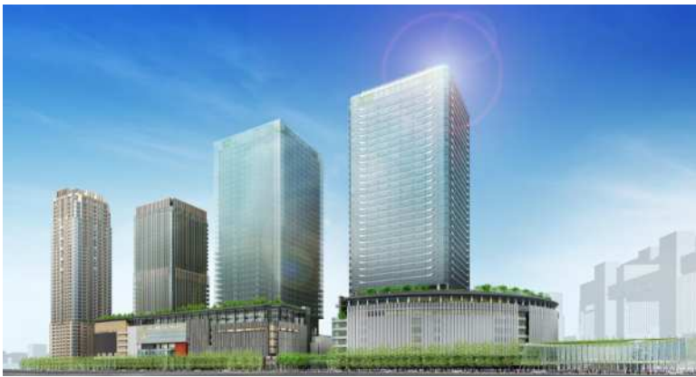
Osaka Station North District
